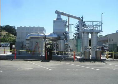
1.4 MW plant at a municipal building
