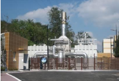
2.4 MW plant owned by an independent power producer
