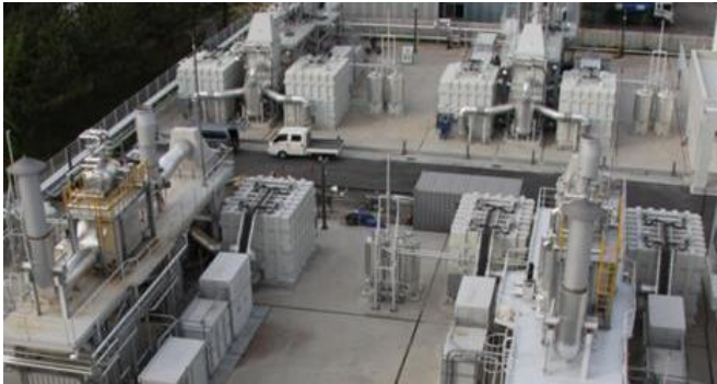
11.2 MW Plant (Daegu City, S. Korea)
