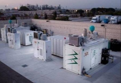
600 kW plant at a food processor
