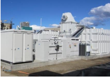
2.8 MW DFC3000 Wastewater Treatment Plant
